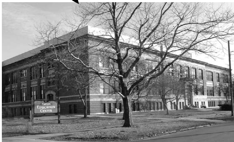
Original site of the Fulton Education Center
