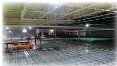
February 2012 — Second floor construction underway.
