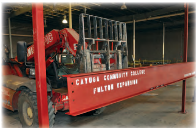
December 2011 — The College held an event called "Building for Growth: Fulton Campus Transformation." It marked the construction kick-off at the River Glen Plaza. Local and college dignitaries and guests were given an opportunity to sign a structural beam within the new 82,000 square foot facility.
